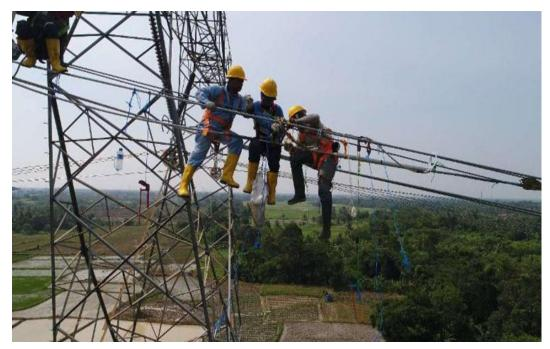
With the support of contractor PT Central Multi Elektrindo, PLN completed a ACCC Conductor upgrade in Indonesia: quad-bundled 500 kV Suralaya — Balaraja ACCC conductor transmission line in West Java near Jakarta.
