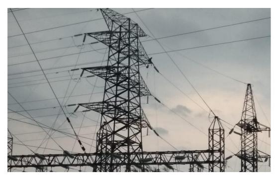
With the support of Power Construction Company One, Vietnam Electricity (EVN) completed their 25 kilometer, 110 KV Phu Lam to Long An, ACCC Reconductor project. EVN selected Glasgow size ACCC conductor supplied by PT KMI Wire and Cable Tbk to replace 240/32 ACSR conductor. Hardware for the project was supplied by PLP.
